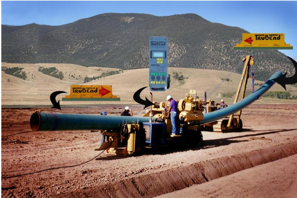
**Place the pipe in the bending machine positioned for the first pull. Clean metal particles from the magnets before placing the transmitters on the pipe. Place one transmitter on each end of the pipe with the arrows pointing toward the bending machine. The transmitters must be on top center of the pipe. Turning the transmitters up right will switch them on. Turning the transmitters upside down will turn them off. Either transmitter may be used at either end of the pipe.**
